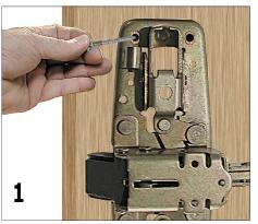
1. Existing Installation: Remove Exit device from door.
